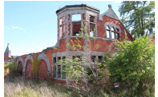
The burned-out shell of the Lockport RR station
