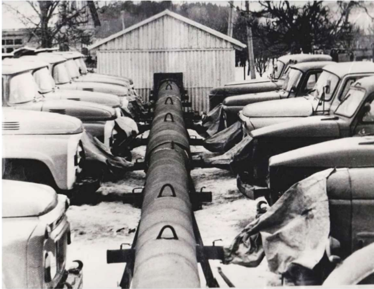
Before block heaters
